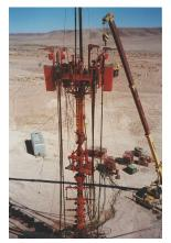
Tubing was snubbed in the well for a controlled circulation kill
